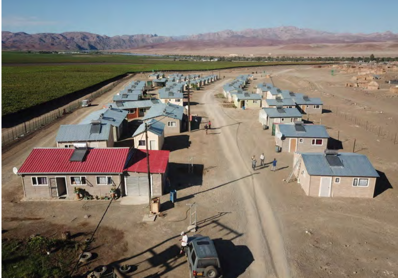
NOBLE PROJECT ... The Orange River Vineyards Investment (ORVI) social housing project which is this year's the winner of the International Energy Agency Solar Heating and Cooling Programme Solar Award
