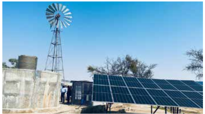
ACCESS TO SAFE DRINKING WATER ... One of the solar powered reverse osmosis units installed by EIF at the three community water points in the Spitzkoppe area.
