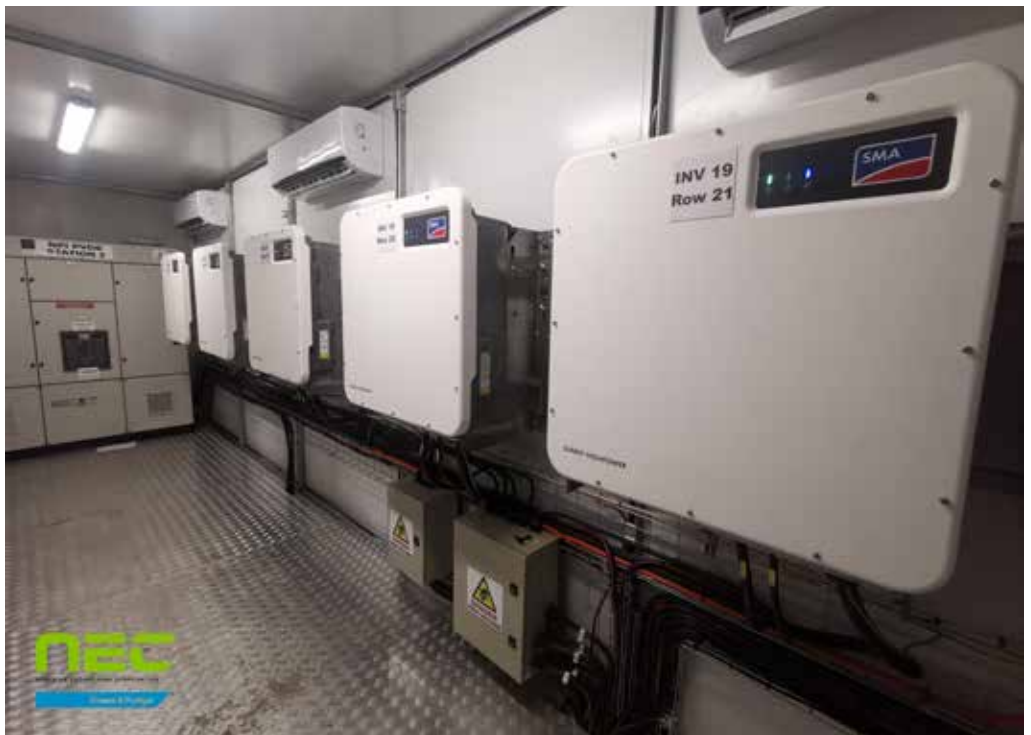
HI-TECH... The solar park's inverter container.
